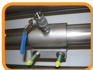
Spot drilling collar
