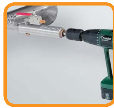
Drilling under pressure with CS drilling jig
