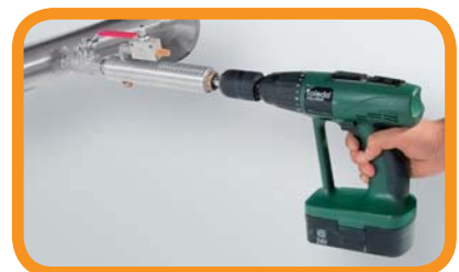
Drilling under pressure
